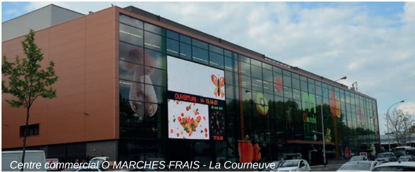
Centre commercial O MARCHES FRAIS - La Courneuve
